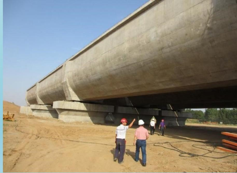
Duan he flum, length 1030m, discharge  $350\text{m}^3/\text{s}$ , increase discharge  $420\text{m}^3/\text{s}$
