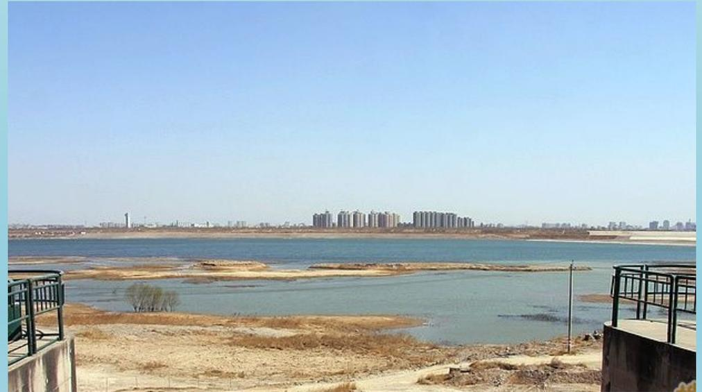
The function of Daning reservoir is regulating water quantity, storage capacity 37 million m<sup>3</sup>, total area 1.34km<sup>2</sup>,
